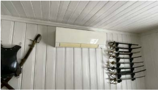
Varmepumpe, innvendig aggregat.
