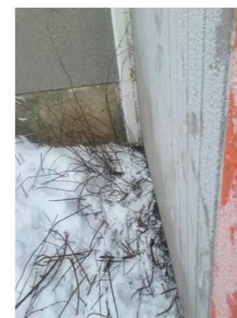
Bakside montert netting
