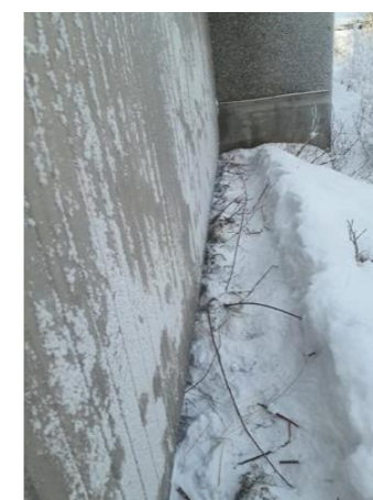
Bakside montert netting
