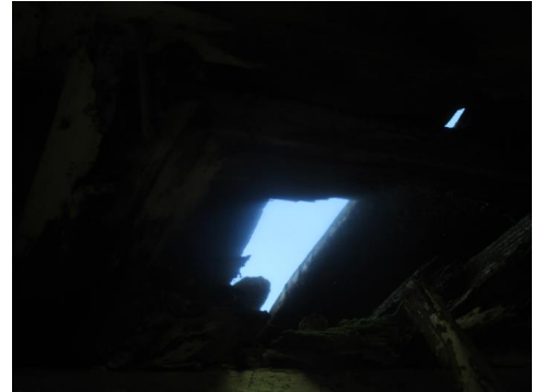
Hull i yttertaket.
