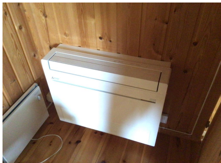
Varmepumpe innerdel.
