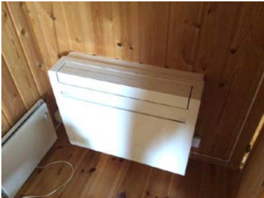
Varmepumpe innerdel.
