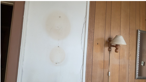
Sprekker i pipe.
