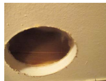
Hulltaking i underliggende himling.
