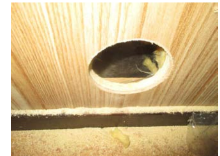
Hulltaking i utfored vegg under trapp.
