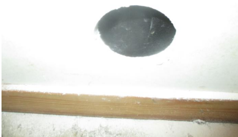
Hulltaking i utfored vegg i bod under trapp.
