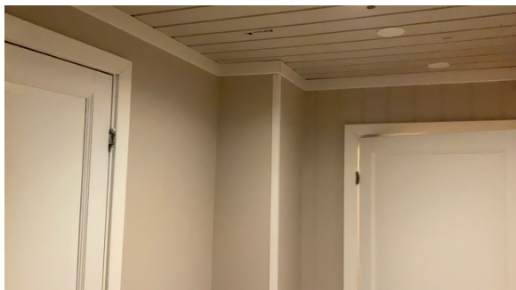
Stakeluke bak innkassing.
