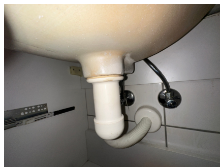
Røropplegg under servant
