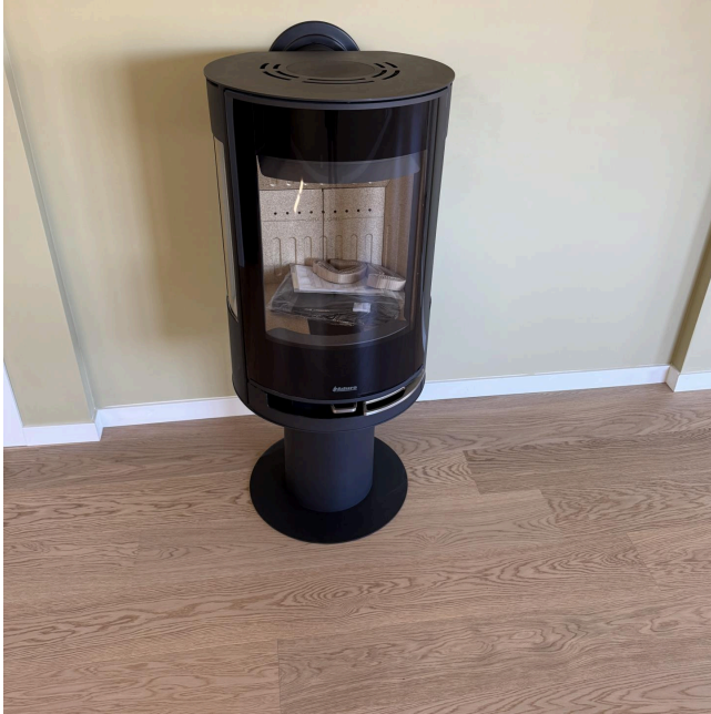
Mangler plate foran ovn.
