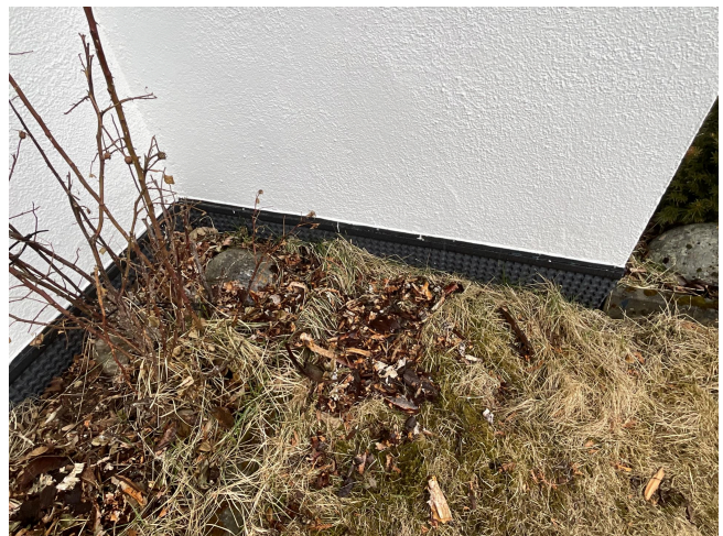
Fuktsikring over hele
