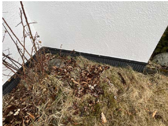
Fuktsikring over hele
