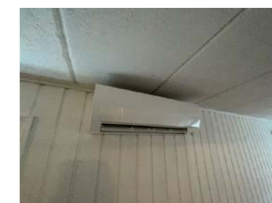
Varmepumpe innerdel.
