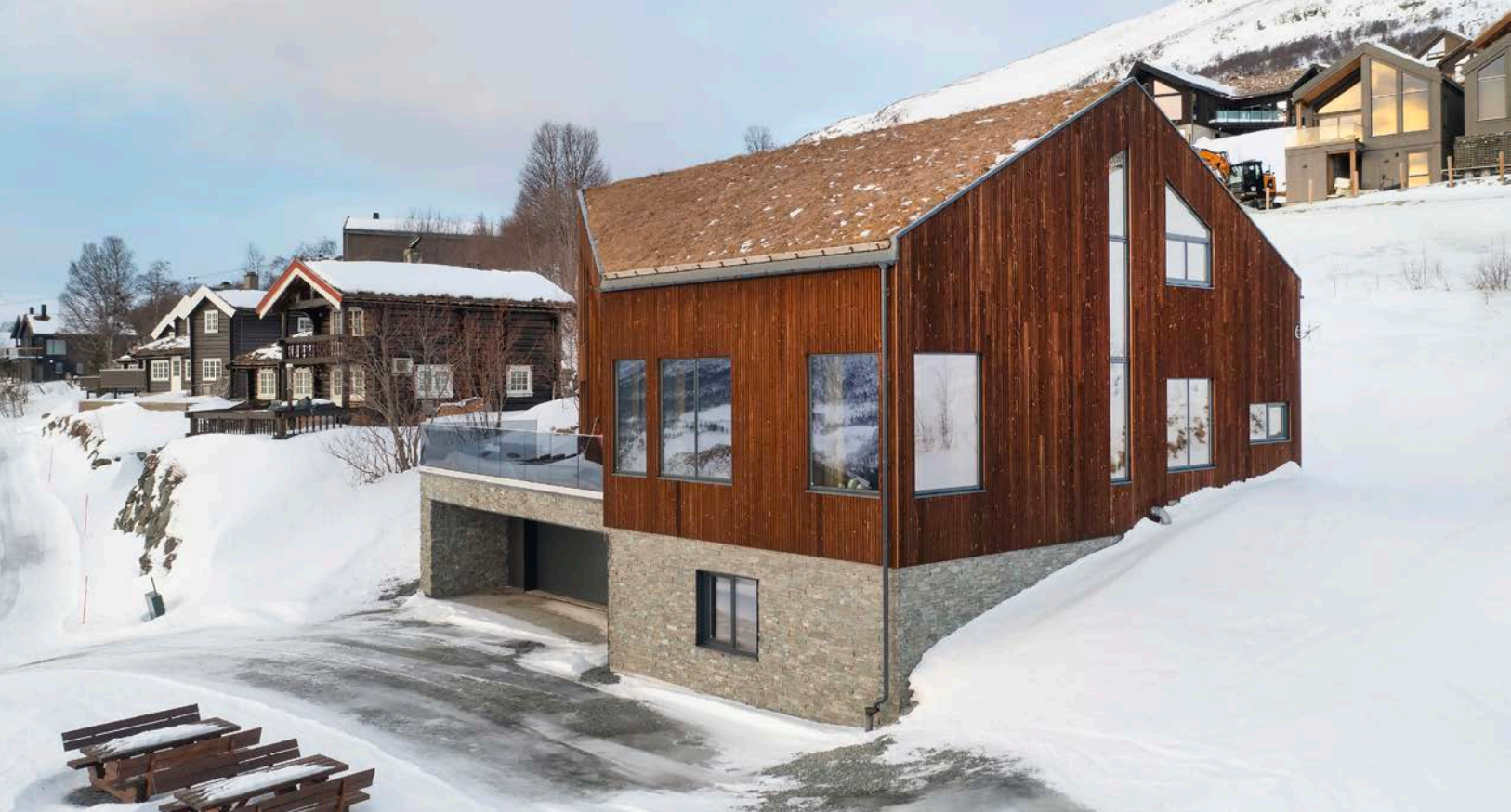
Fasade - store glassflater
