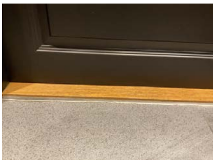
Manglende tilluft bad.
