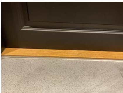
Manglende tilluft bad.
