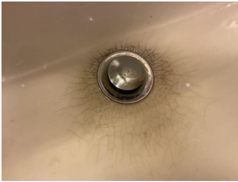
Riss/sprekker i servant.
