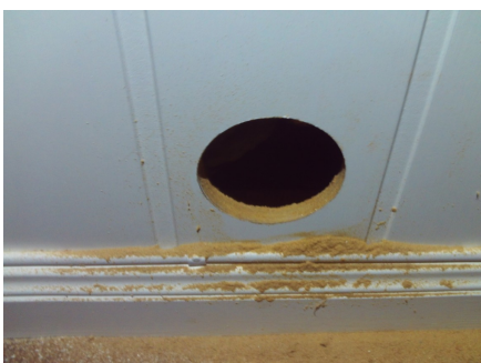
Hulltaking i utfored vegg.
