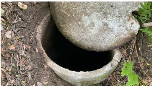
Slamavskiller i betong.
