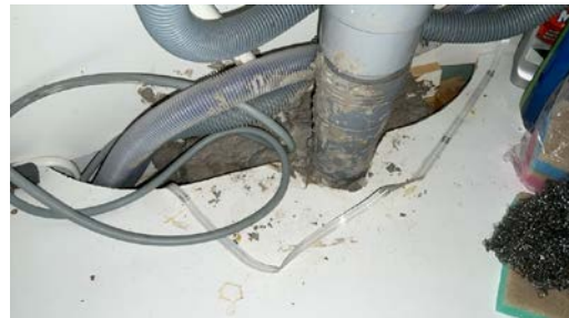
Betongtetting for mus
