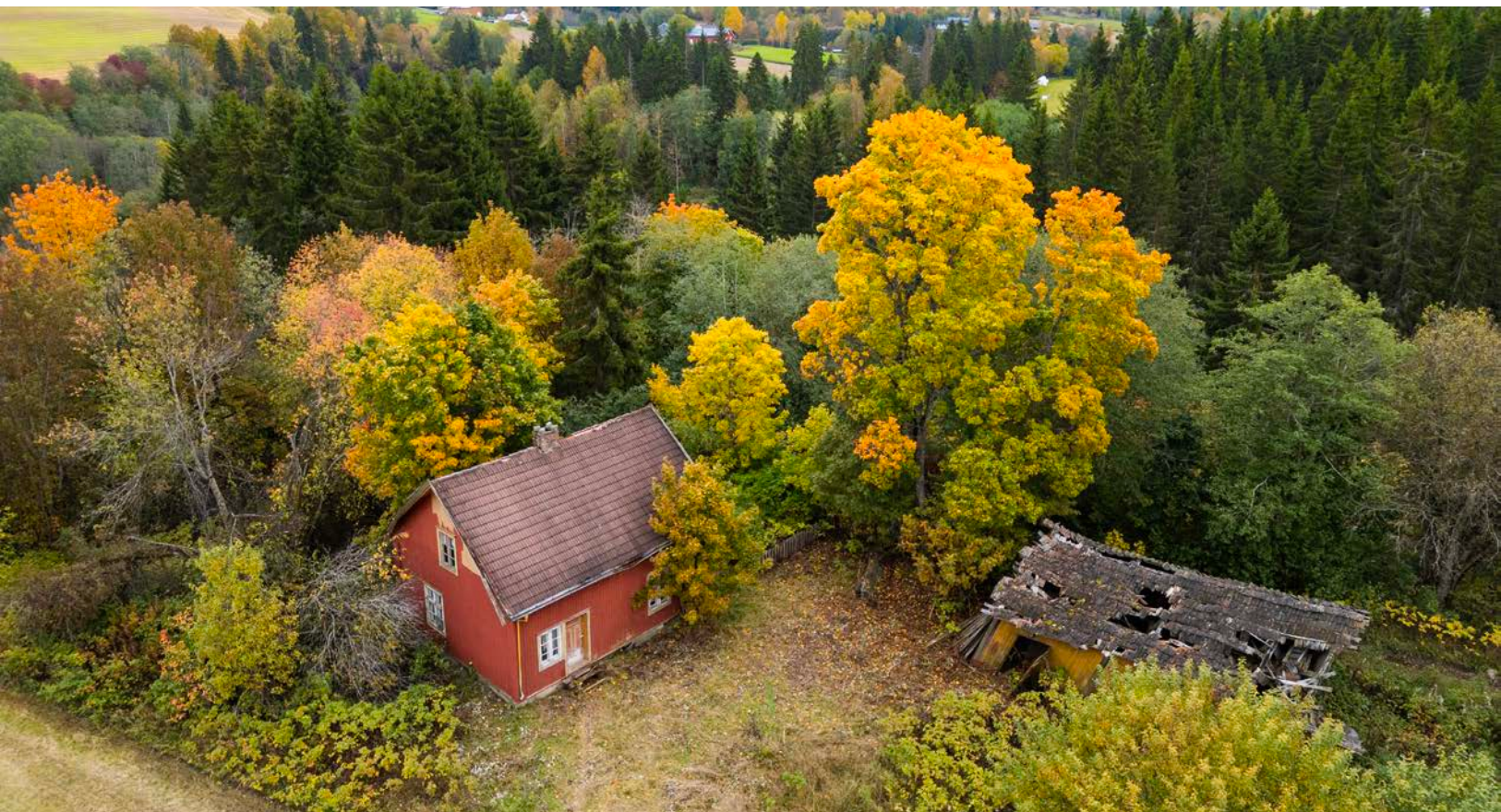
Behov for oppgraderinger.
