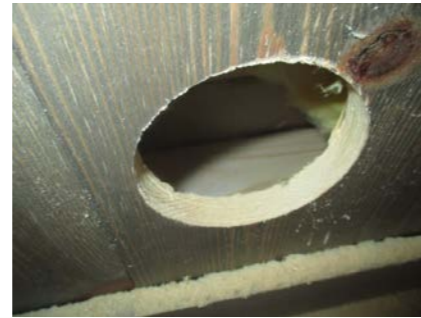
Hulltaking under trapp.
