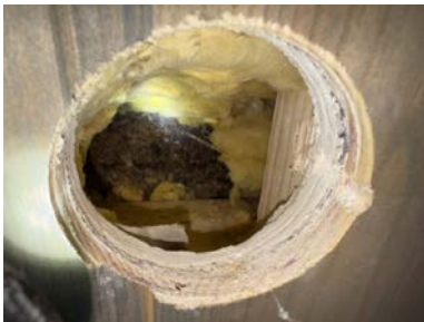
Hulltaking i bod under terreng
