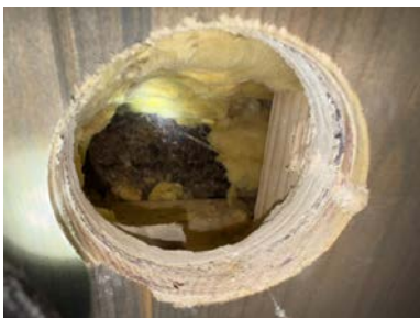
Hulltaking i bod under terreng
