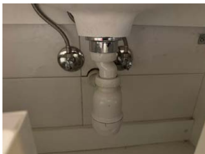
Røropplegg under servant.
