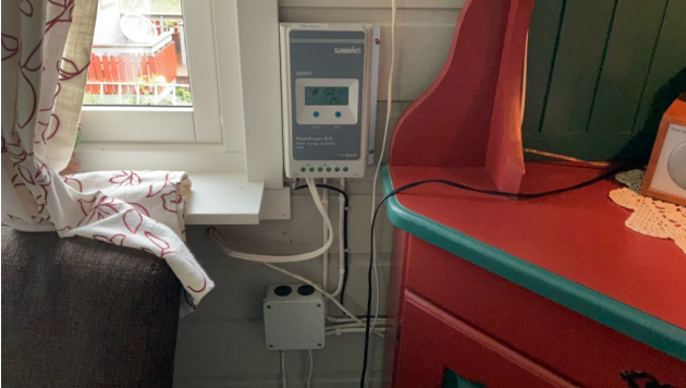
Styringspanel for solcellepanel.
