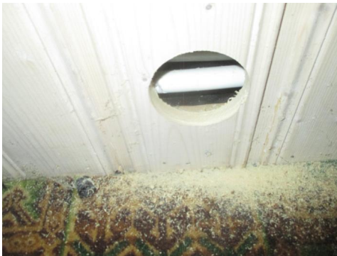
Hulltaking under trapp.
