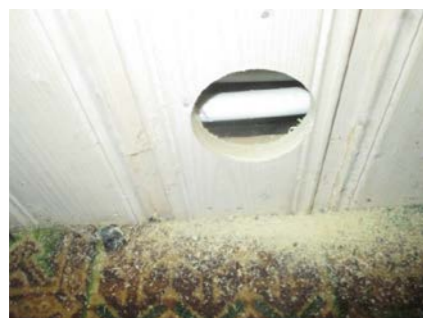
Hulltaking under trapp.
