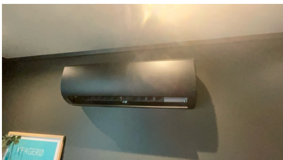
Varmepumpe innerdel.
