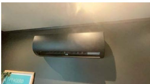
Varmepumpe innerdel.
