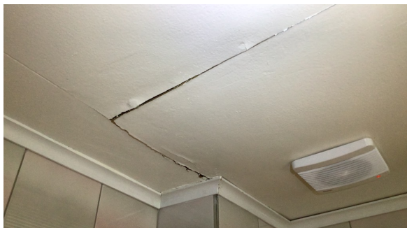
Fuktskadet himling.
