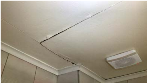
Fuktskadet himling.
