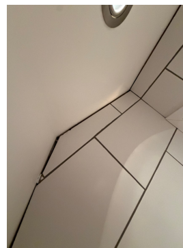
LOFT > BAD/VASKEROM - 3.2M2
