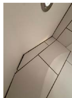
LOFT > BAD/VASKEROM - 3.2M2
