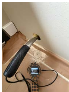
LOFT > BAD/VASKEROM - 3.2M2
