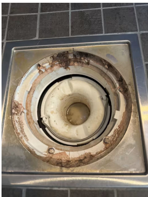
Membran under klemring.
