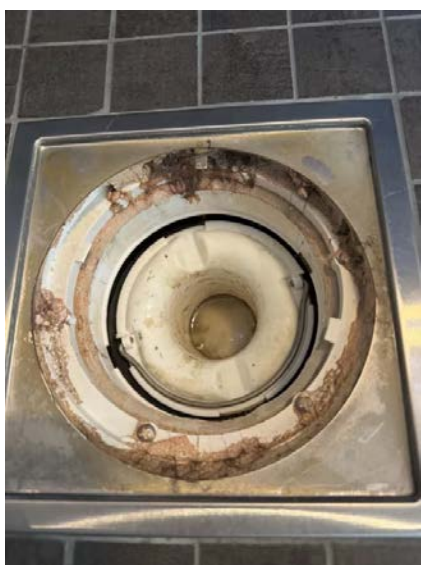
Membran under klemring.
