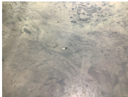
Skadet vinylbelegg.
