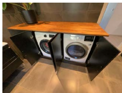
Opplegg for vaskemaskin.
