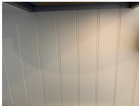
Mdf panel over benkeplate.
