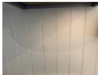
Mdf panel over benkeplate.
