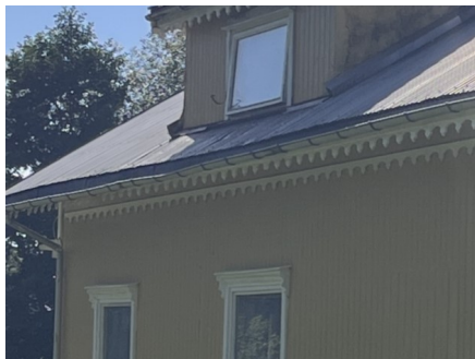
Deformert takrenne.
