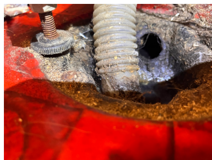
Plugg i sluk mangler.
