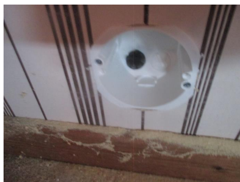
Hulltaking i utfored vegg.
