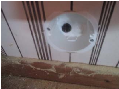
Hulltaking i utfored vegg.
