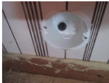
Hulltaking i utfored vegg.
