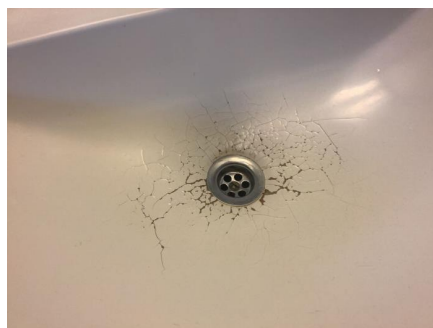
Krakelering i servant.
