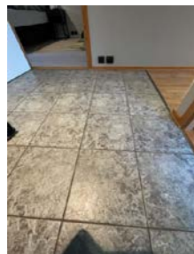
- Riss/sprekker i enkelte flisfuger i gang
