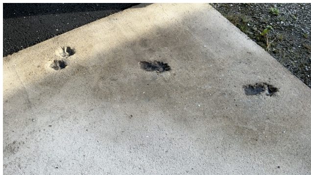
Dekke v/ carport
