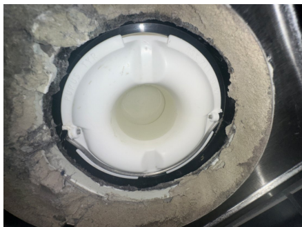
Sluk i plast, plassert under servant
